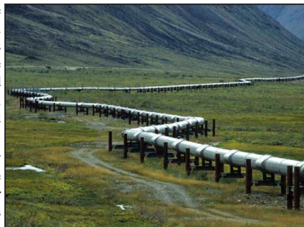
The oil pipeline across the North Slope, so cold that cooling of piles into the permafrost is not needed.
