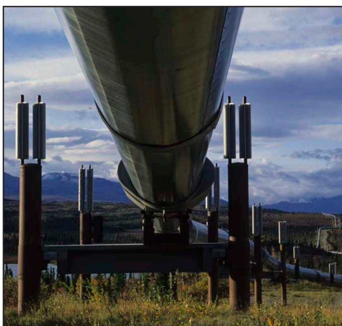
The elevated oil pipeline with cooling fins on the piles to ensure conservation of the permafrost.
